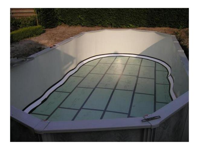
The Styrofoam plates and pool cove are in place. As mentioned earlier, it's also possible to lay these plates entirely underneath the pool.
