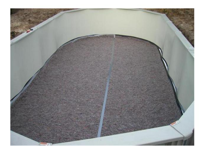
Whether there are isolation (foam)plates, a sand or concrete floor under the pool, it is always best to use an underlayment (sort of carpet) before mounting the liner. It is protective and takes away any (left behind) little unevenness.
