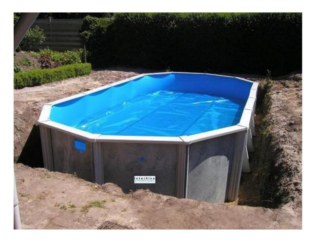
On this picture mounting the liner has been finished. But you can only start finishing the liner when there is about 60–70 cm of water in the pool. Not sooner, because the liner may shift a little during the filling process.
